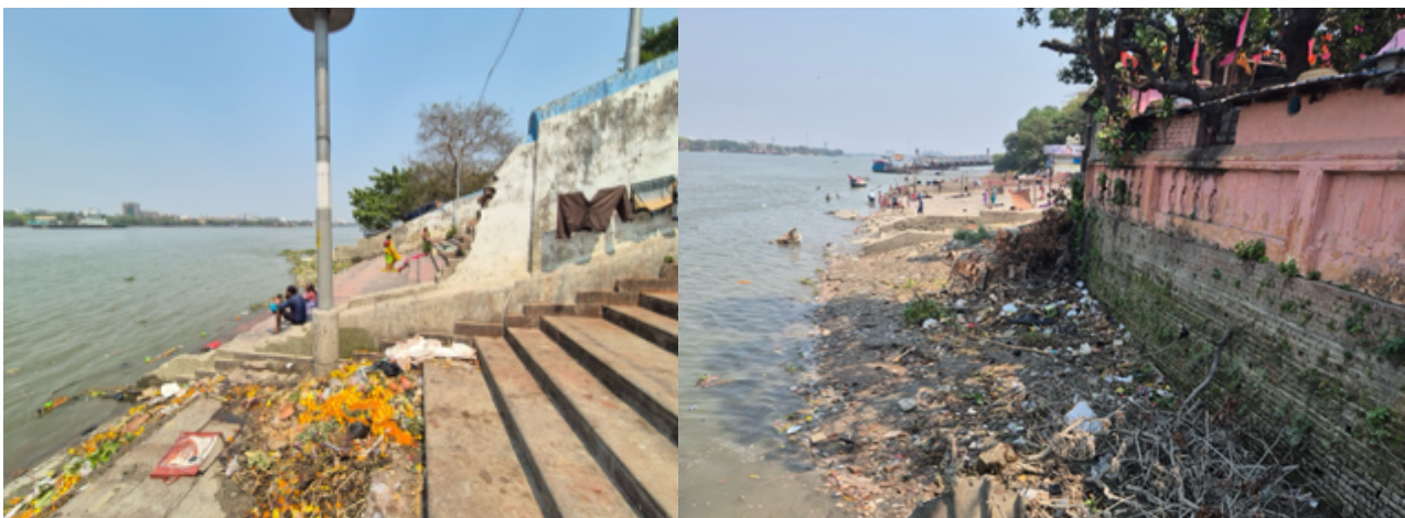
Existing condition of the site
