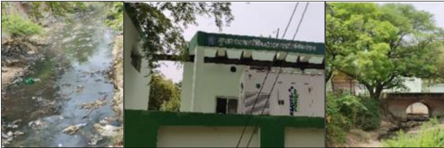
Figure 6: Tapping Station at Guptar Ghat, Kanpur
