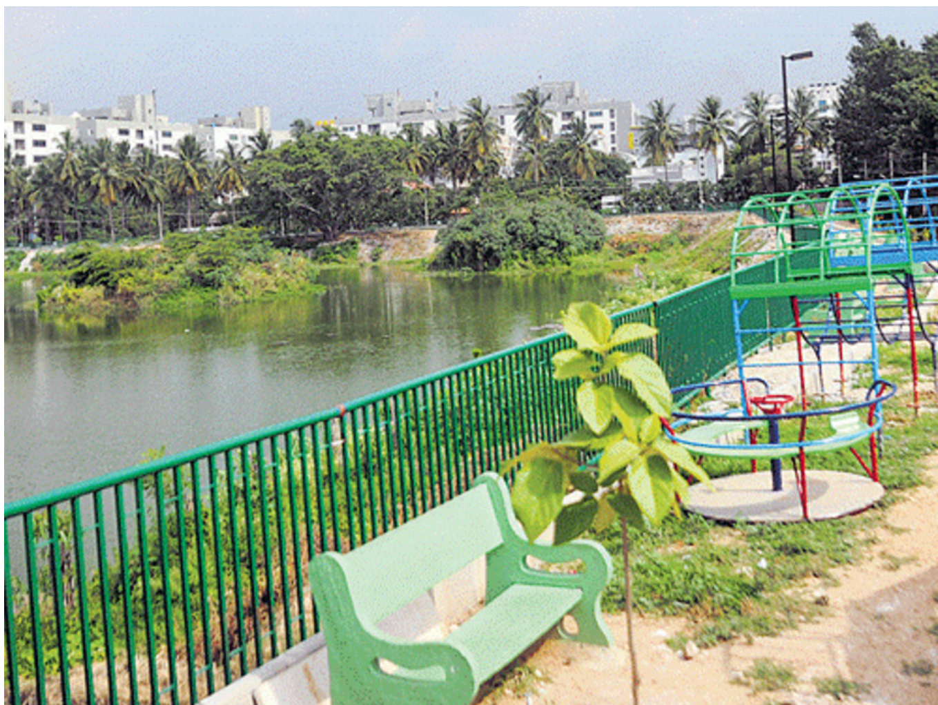
Figure 7: Example of cast iron railing fencing for boundary protection of water bodies
