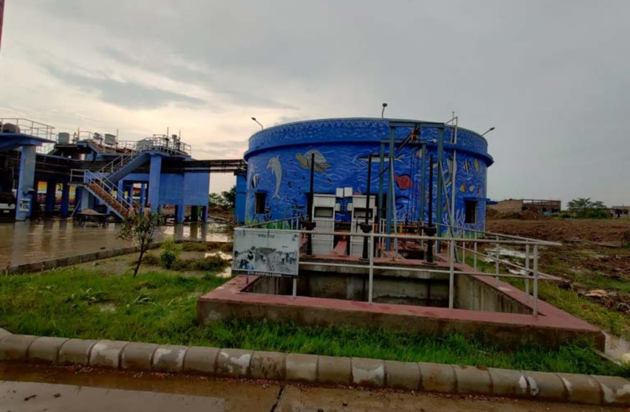
Glimpse of sewage infrastructure under creation in Patna (Source - NMCG)
